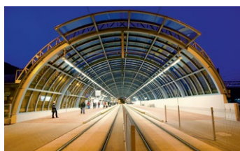
INTEGRATED COMMUNICATION CENTRE POZNAŃ, POLAND
